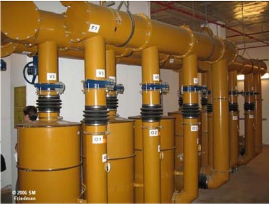
*Closed Air Filtration System for protection against biohazard.*
